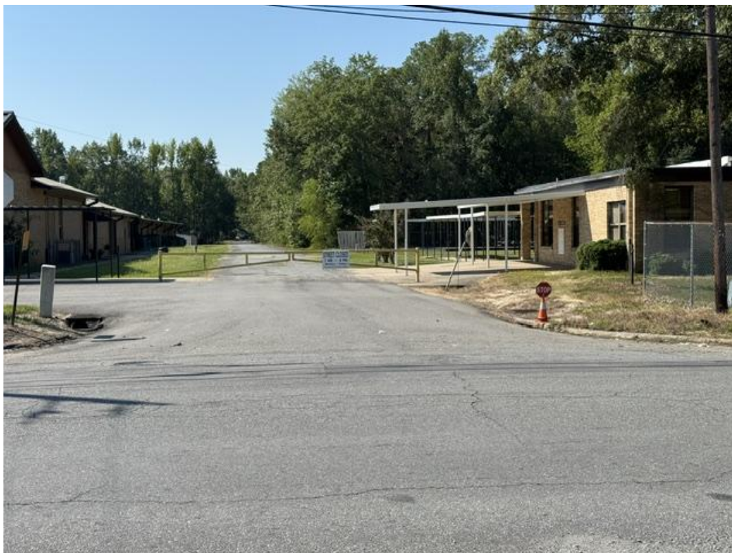
Looking toward area of new cafeteria – between buildings
