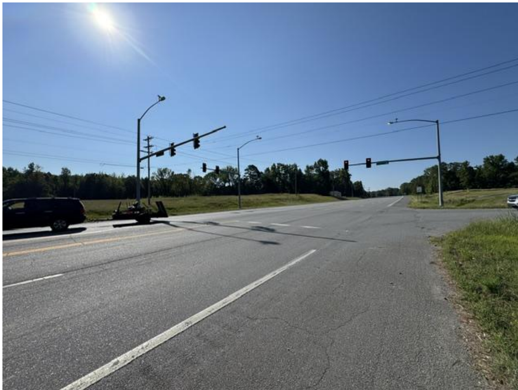
Ridgway & Olive intersection looking south
