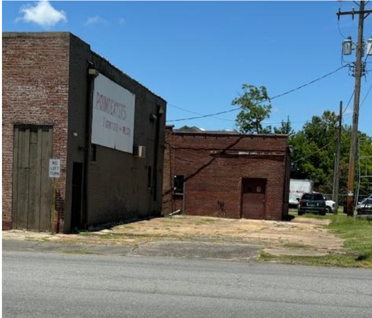
Back of building
