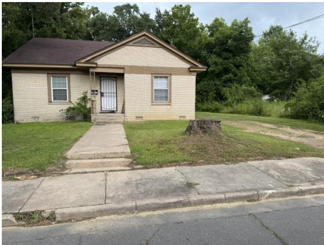
House behind and west of 1306 S. Oak
