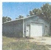
EXISTING STORAGE SHED
