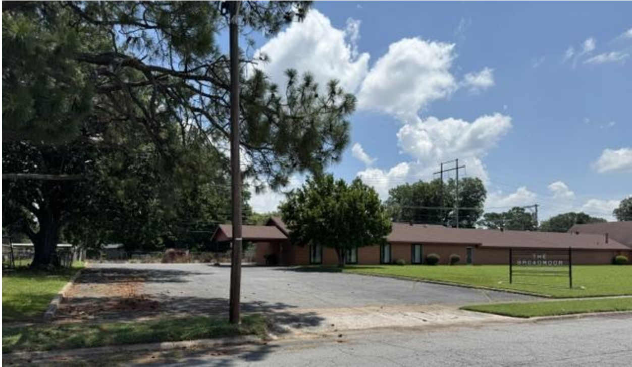
1205 Wisconsin view from north side – parking and building access point
