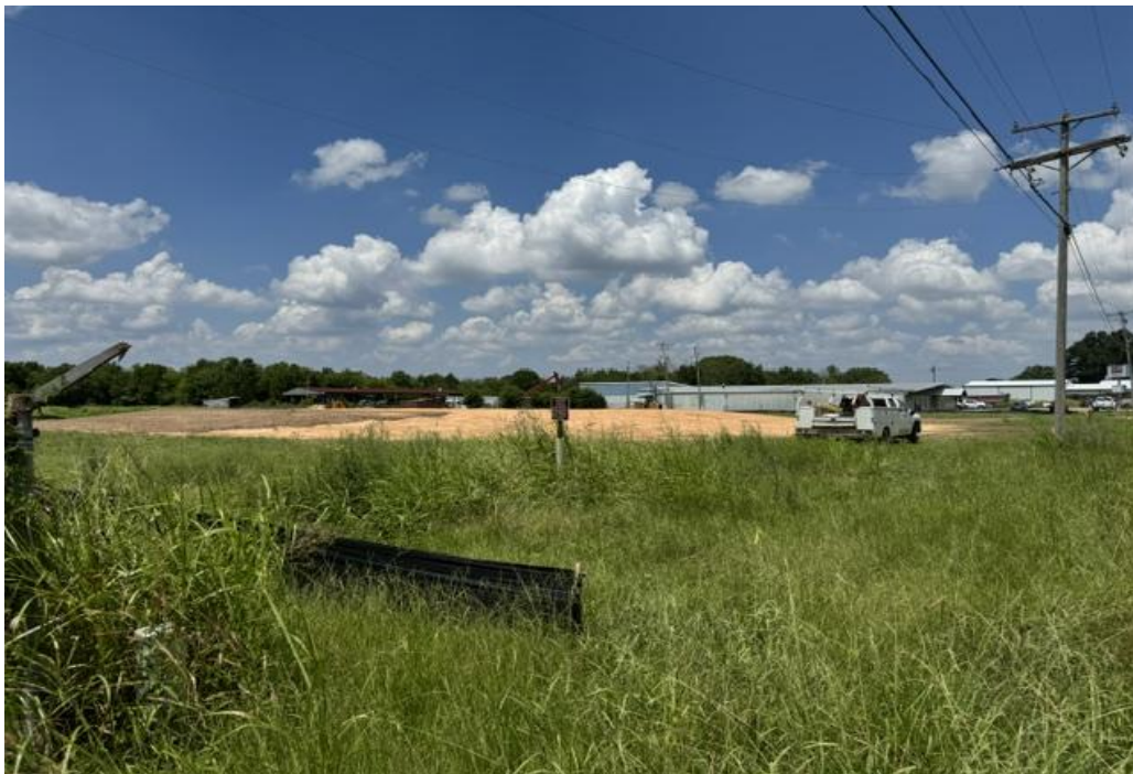
200 Grider Field Ladd Road – site under construction
