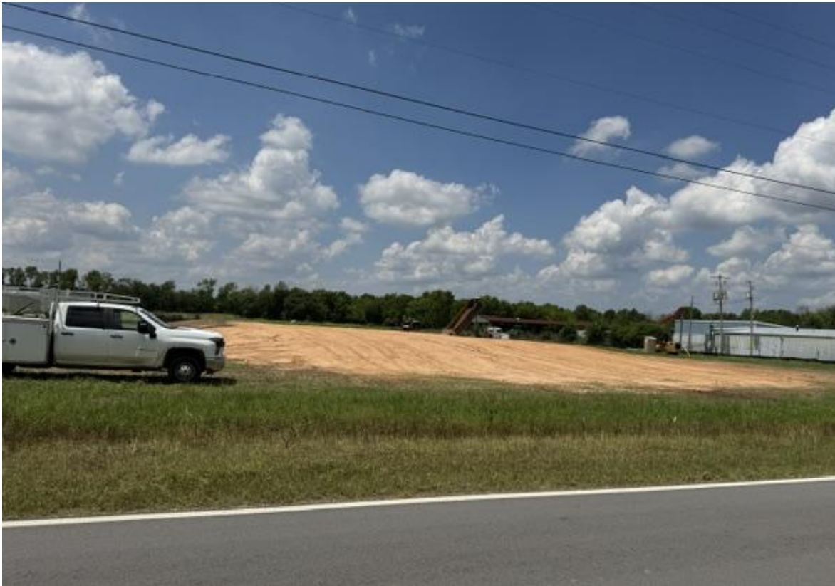
200 Grider Field Ladd Road – site under construction
