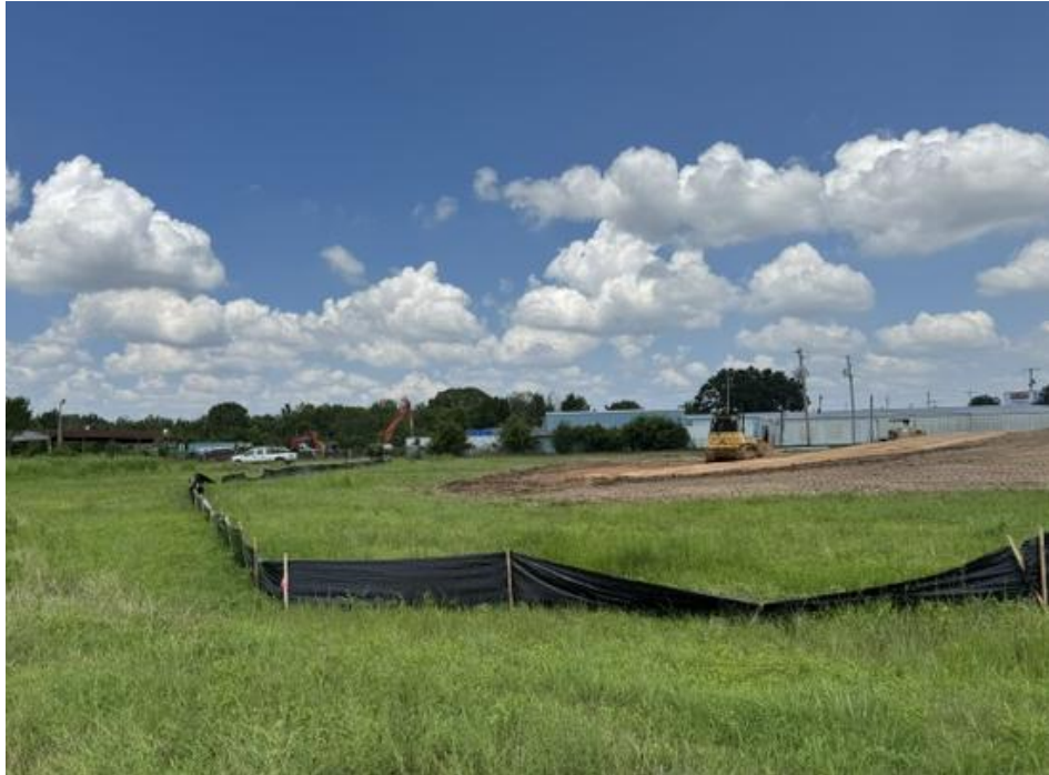
West view of construction site
