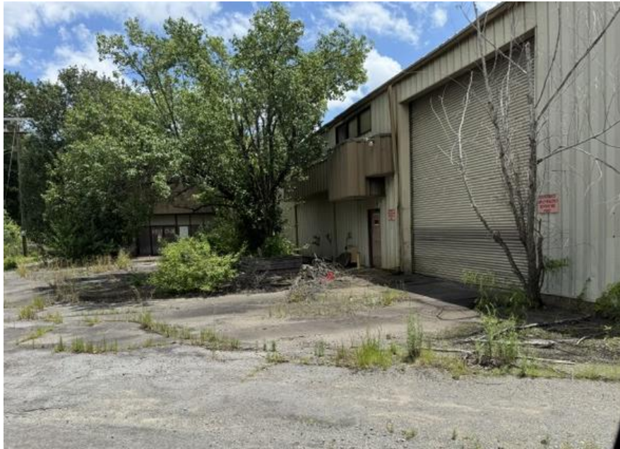
Front of first building – old office area
