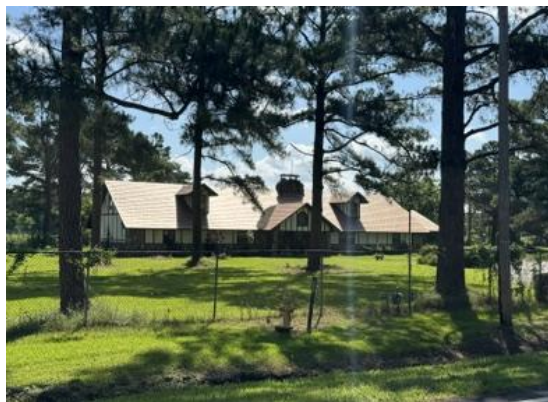
Single family residence south of and adjoining site – closer view
