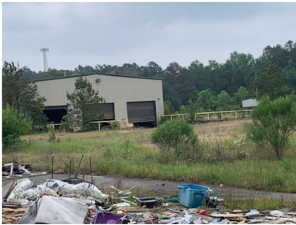
Previous (2025) photos of debris -
