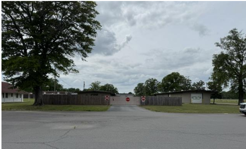
Maintenance structures north of 601 Hangar Row
