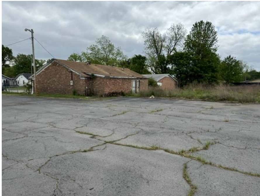
Properties east of rear of 1222 W. 6 th
