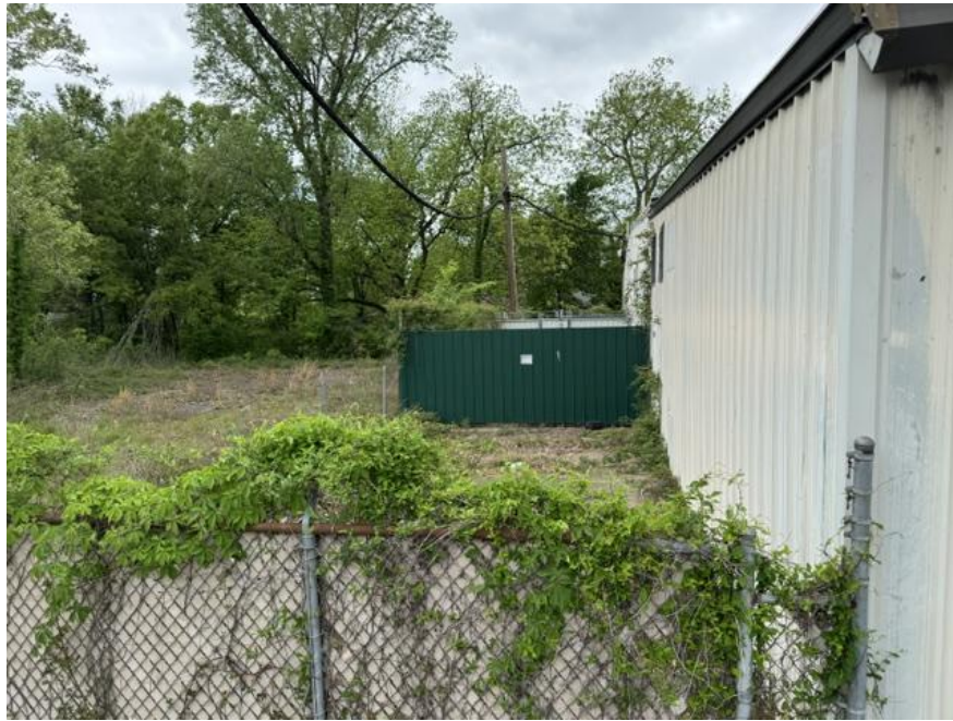
Rear (south) view of 1222 W. 6 th Avenue
