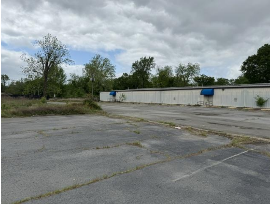
East side of 1222 W. 6 th Avenue
