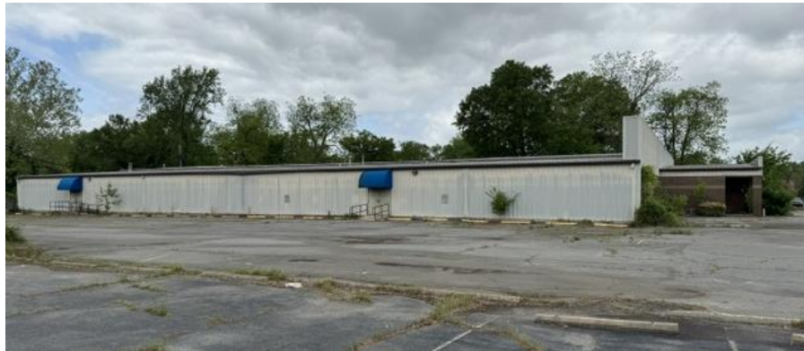
East side of 1222 W. 6 th Avenue
