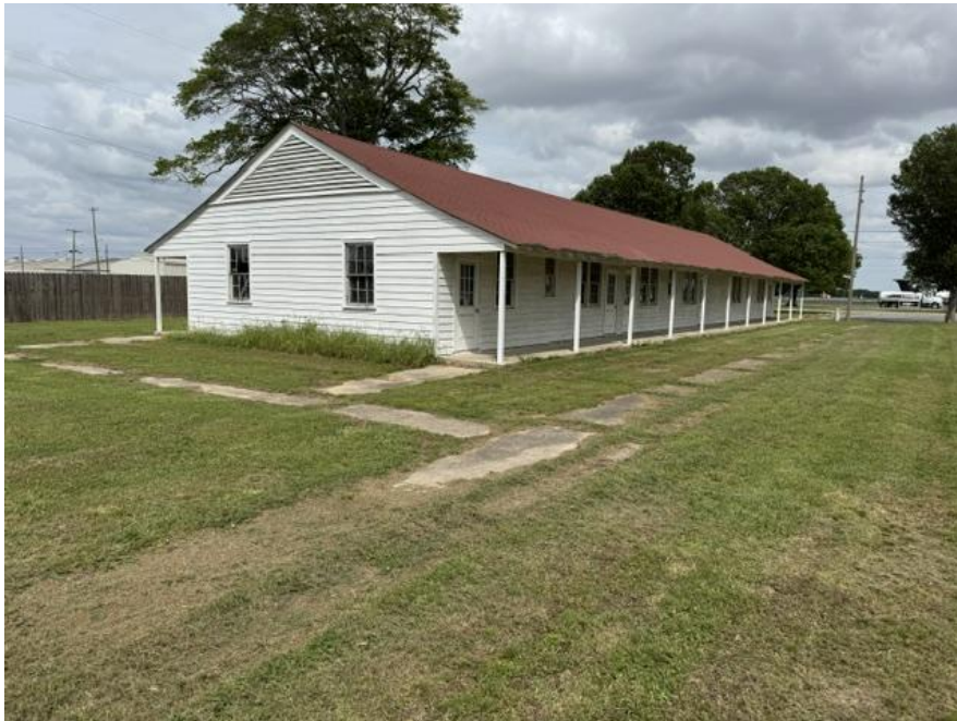
601 Hangar Row – west view
