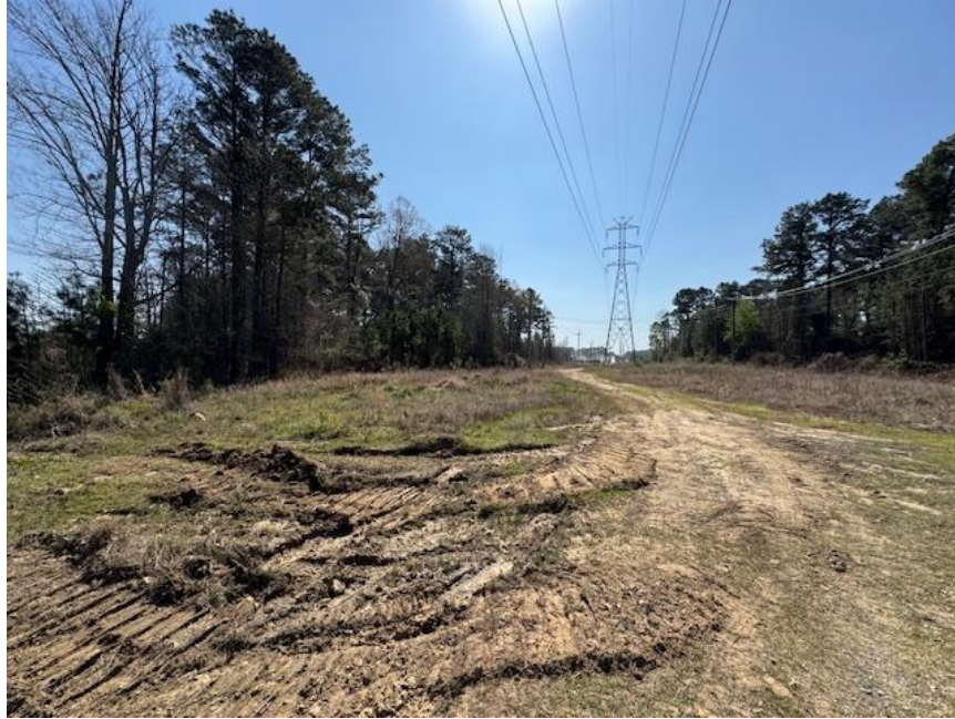
Power line view – looking south toward plant
