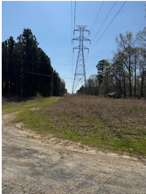
View south down power line from area near cell tower
