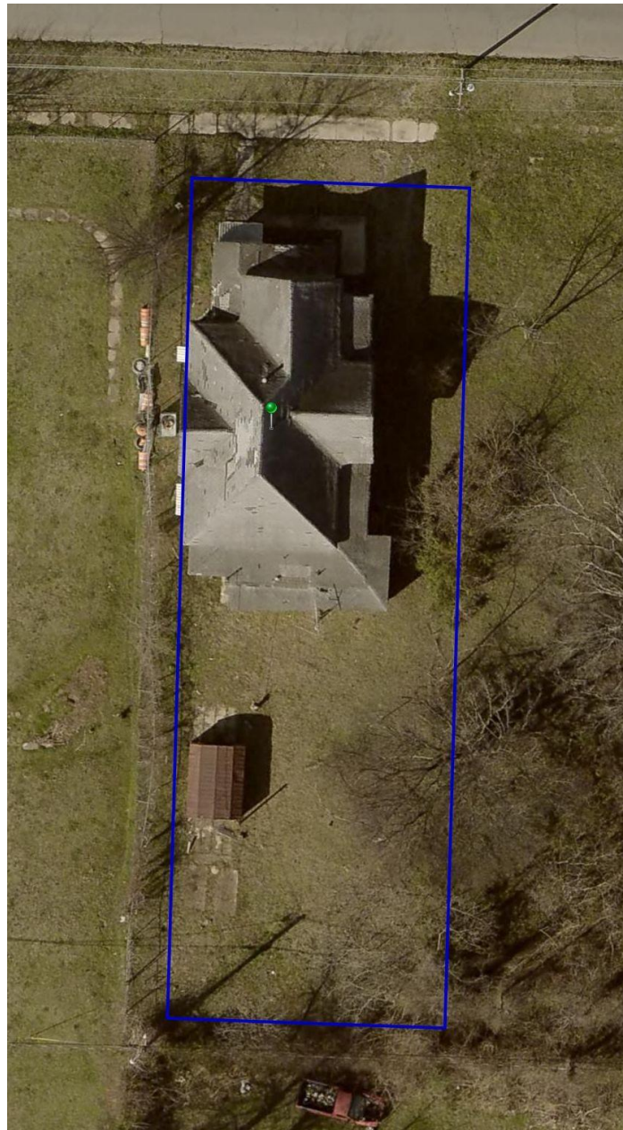
Site view – close up
