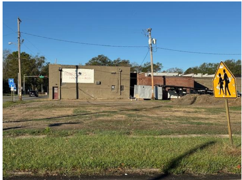
Surface graded. (Photo taken 11-14-24)
