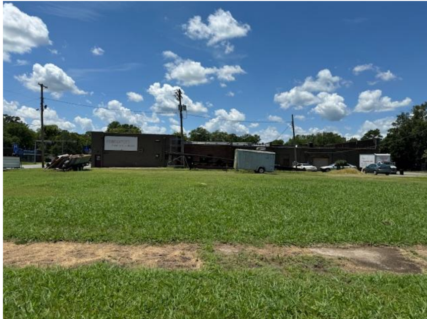
Back side view looking west toward building
