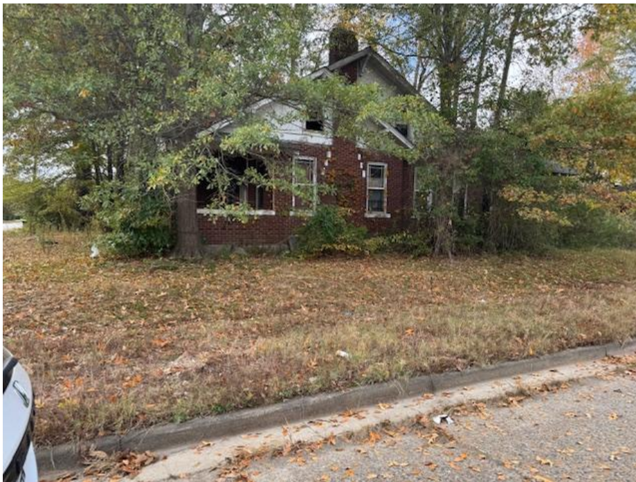
Adjoining property to the east
