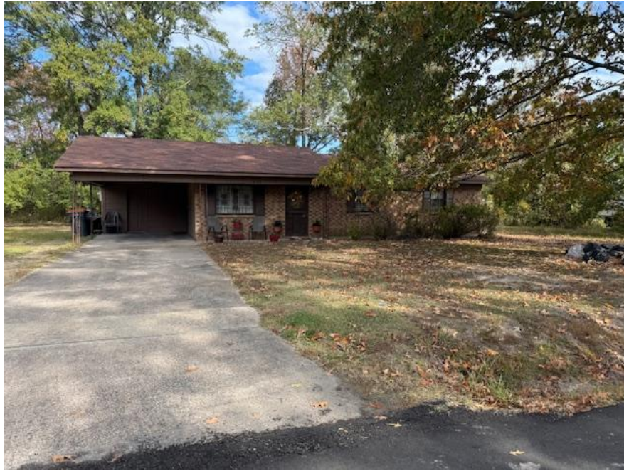
4107 W. 15 th – Adjoining property to west
