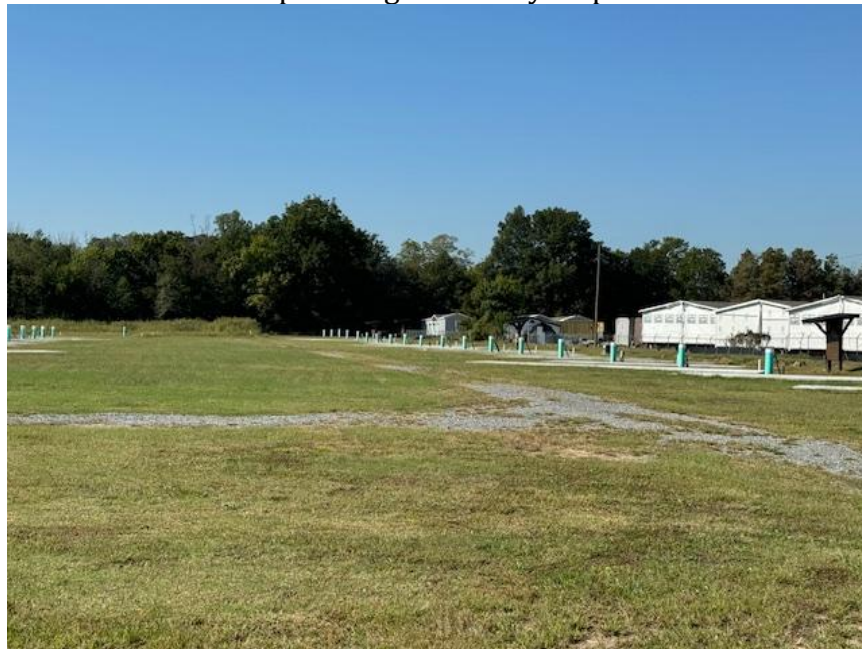
Note RV pad and utility connections in place. Gravel base not yet spread.
