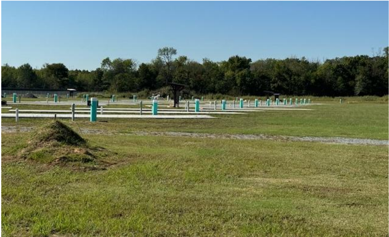
Note RV pad and utility connections in place. Gravel base not yet spread.
