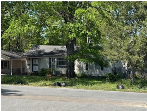
Residence to west
