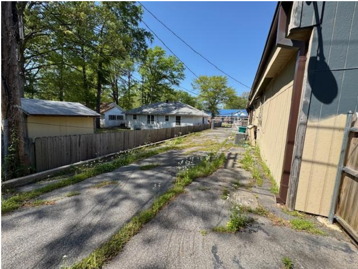
Back side of Retail center
