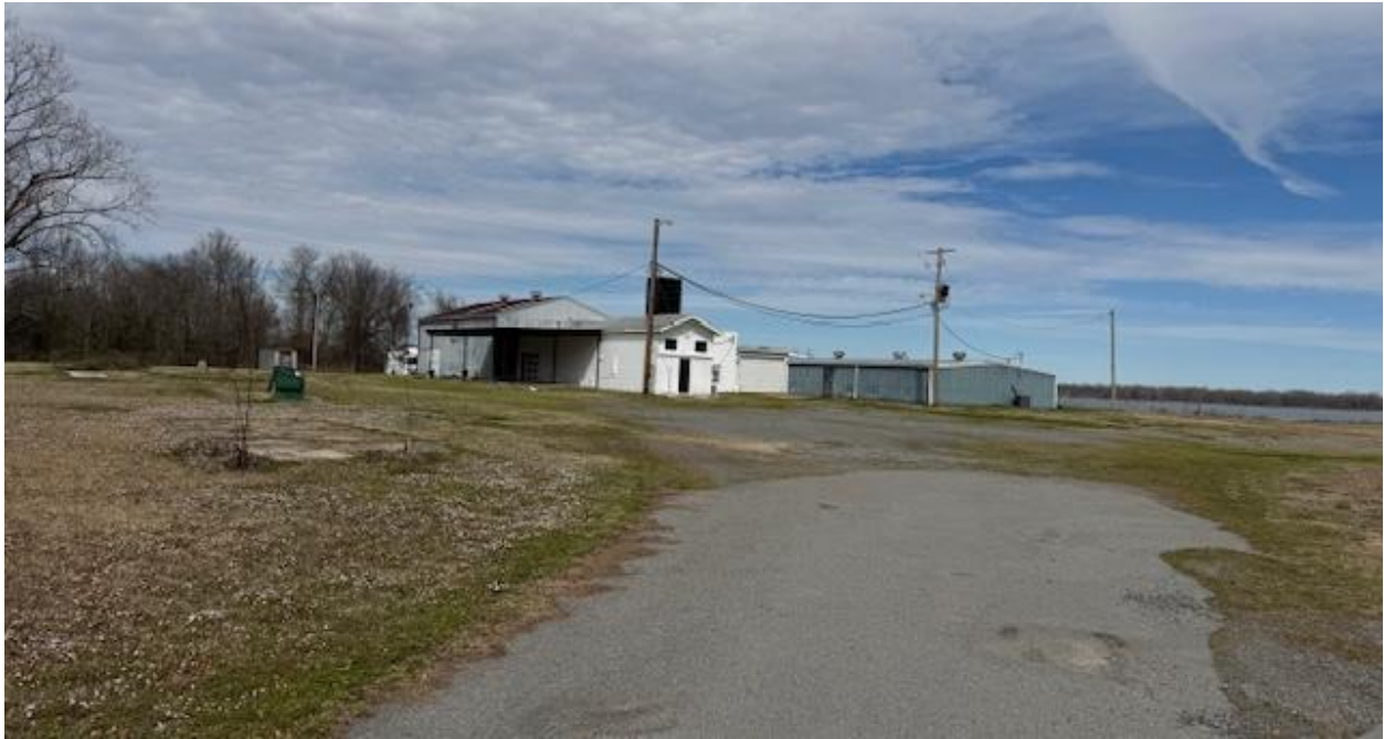
Building view from entrance off Bell and Locust
