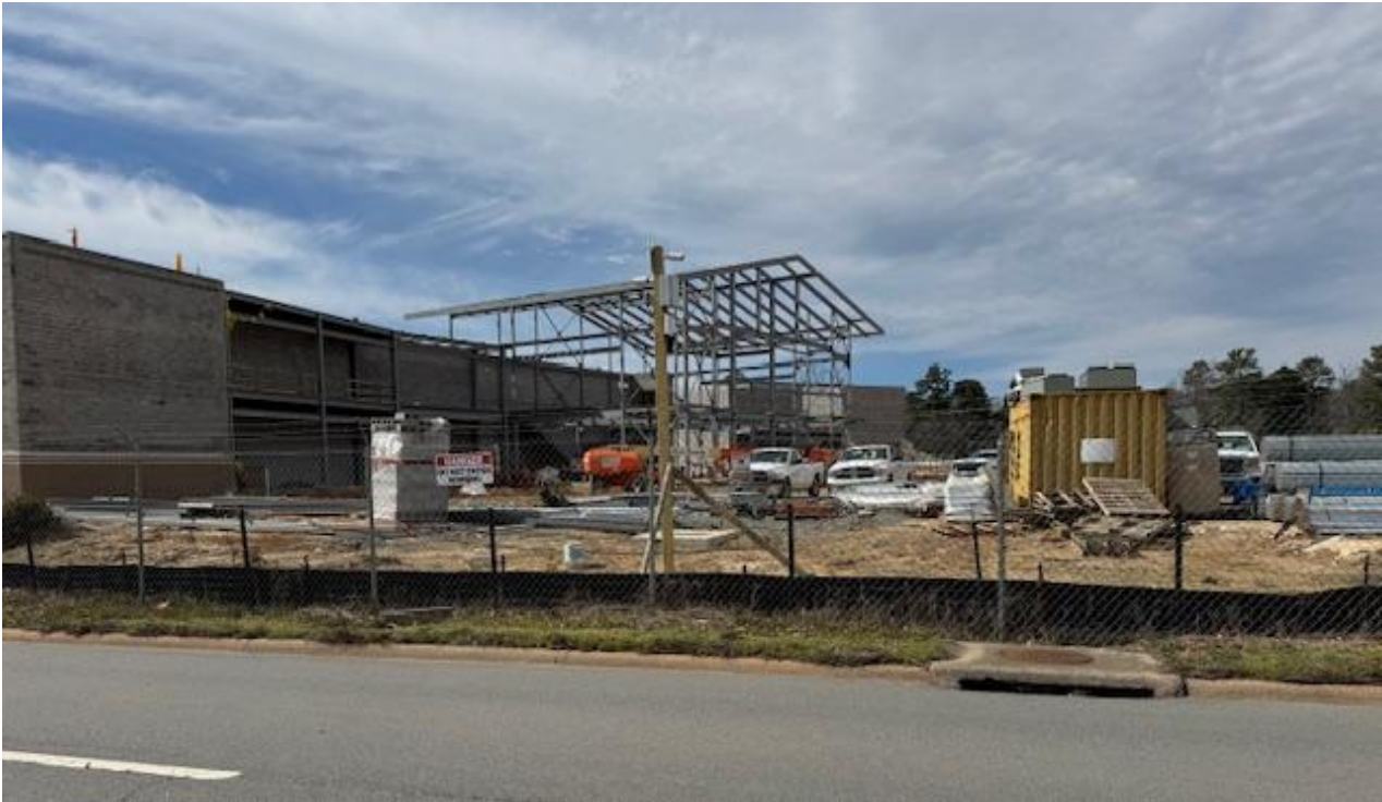
New Construction front view Hwy 79
