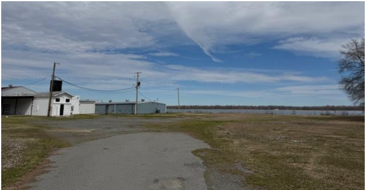
Building view from entrance off Bell and Locust (Lake Saracen in background)
