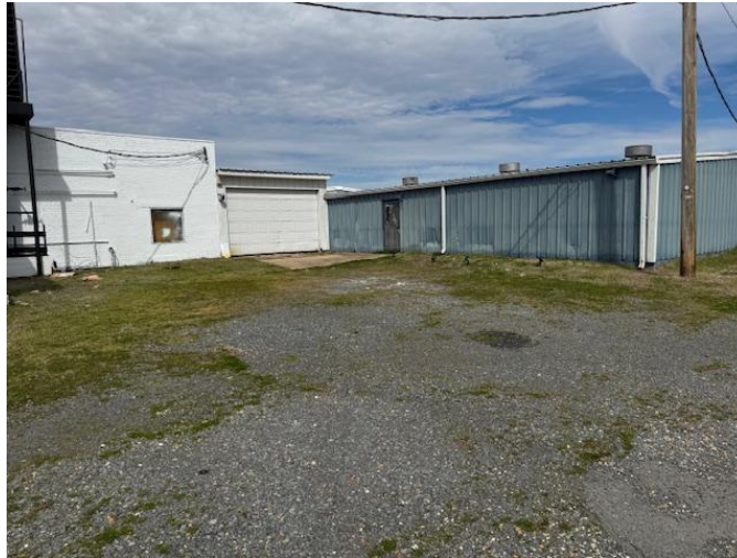
South side of building former primary access
