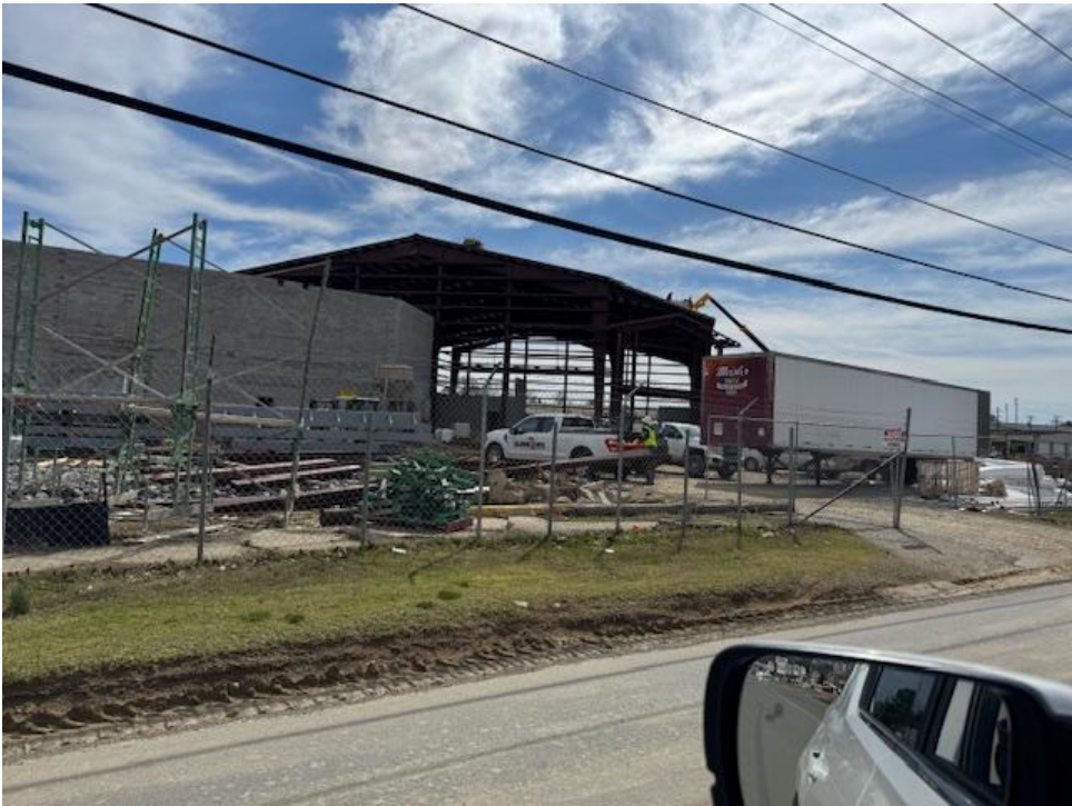
Front looking southwest
