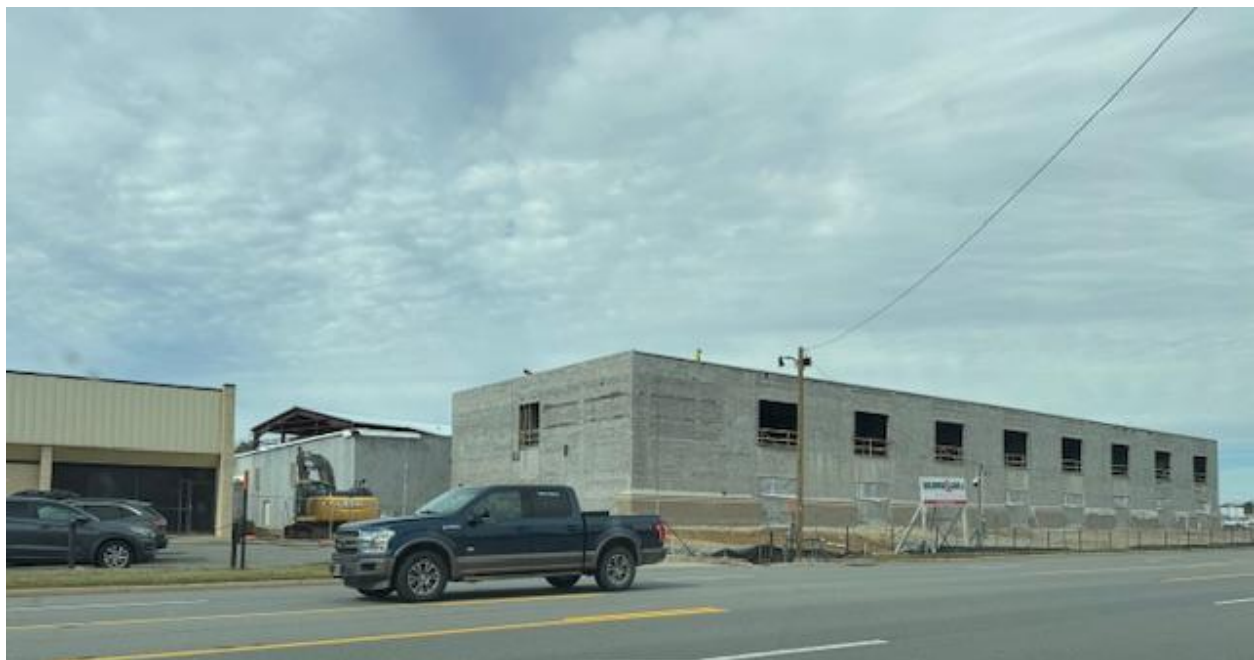
New construction (north along Hwy 79)
