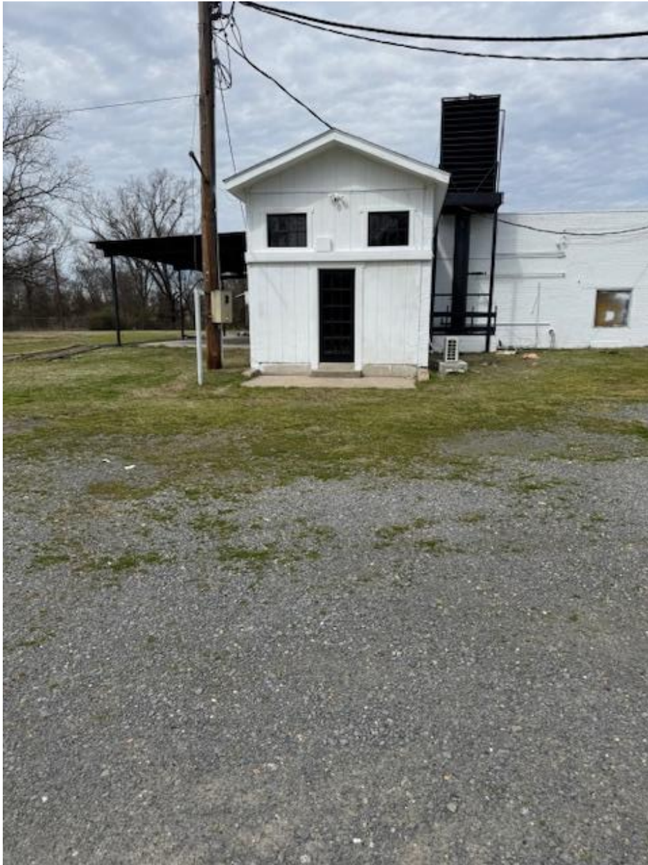
South side of buildings – access point (gravel parking)
