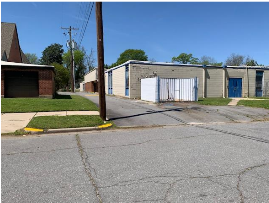
Southeast side of 708 W. 2 nd adjoining Trinity Episcopal Church
