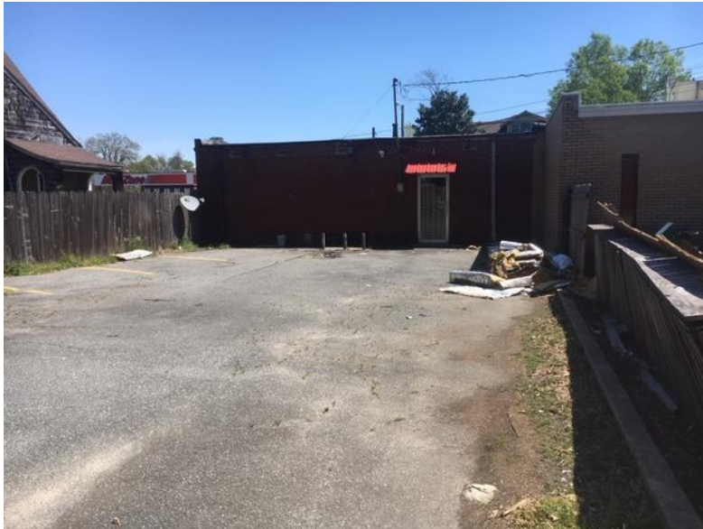
Rear of building
