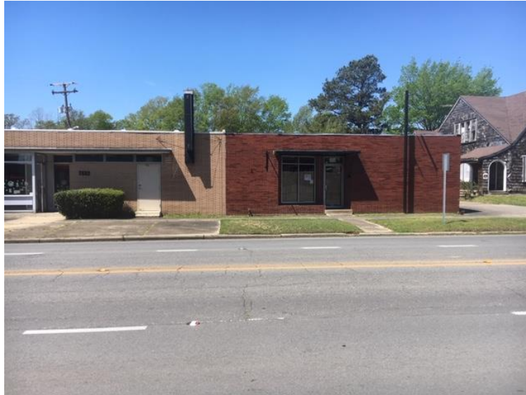
Front of building
