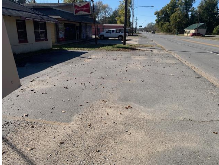
Front view looking west
