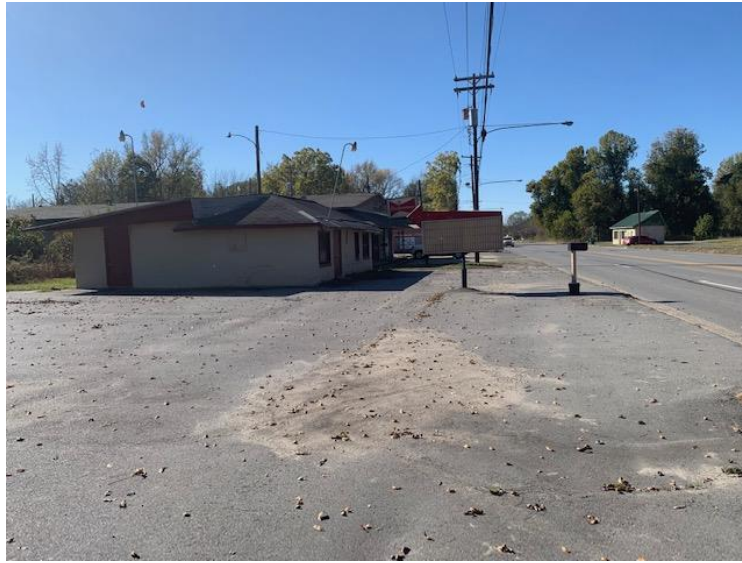
Looking west from east side of building
