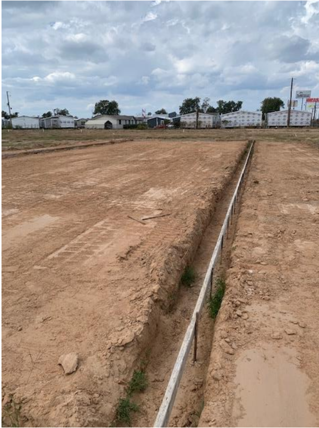
Office site footing
