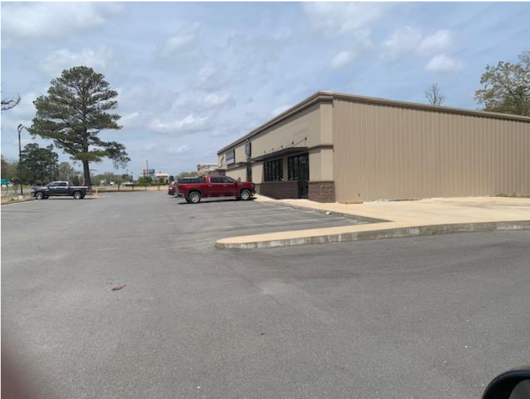
View west (front parking area)
