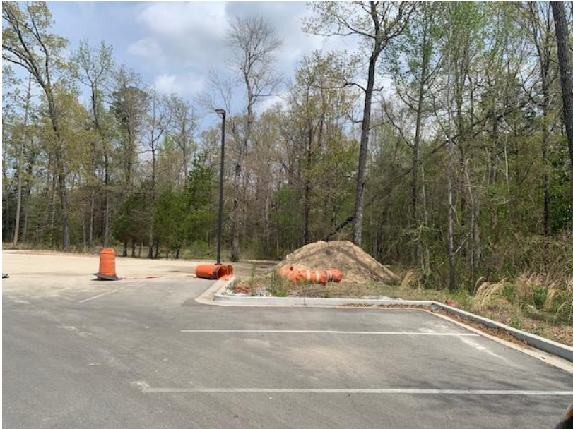
Rear -East side view
