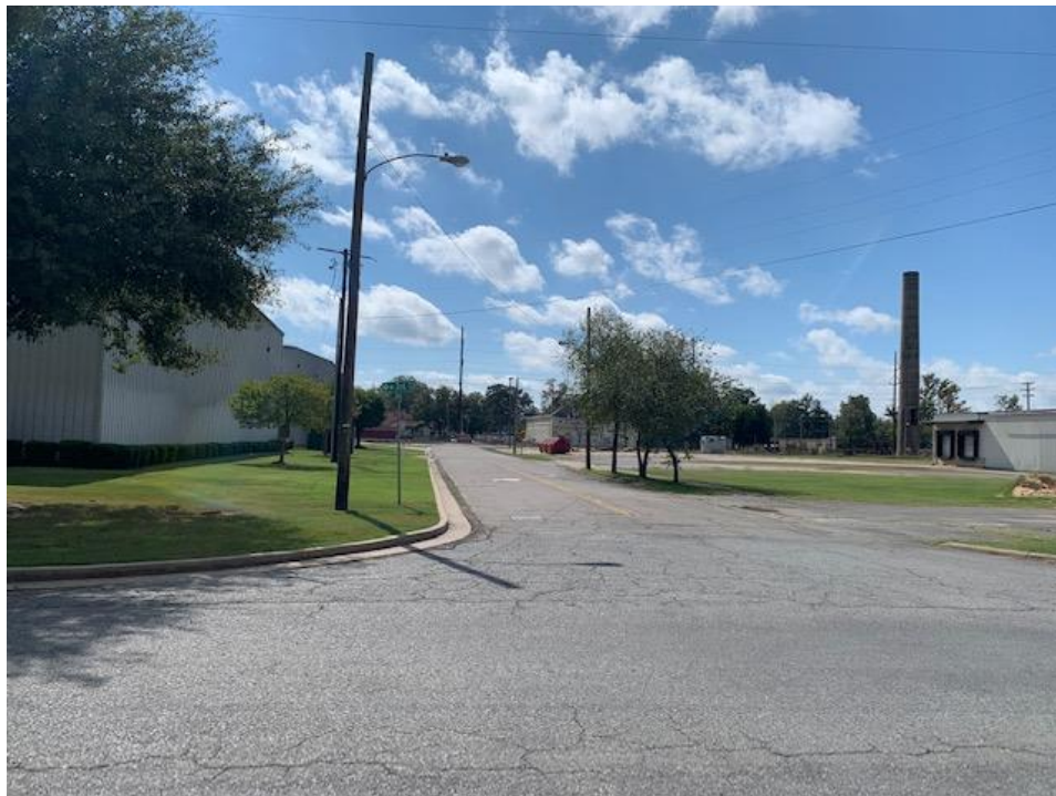
View south down Mulberry
